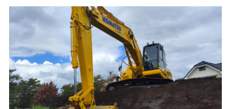
Slope Building in Pond
